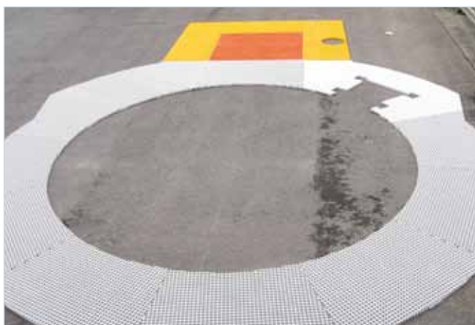
Laying of a platform for testing at the work
