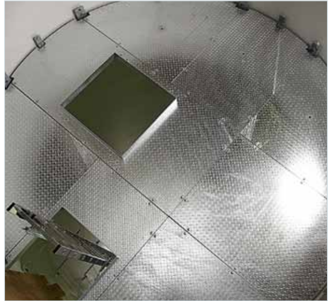
Intermediate platform made from chequer plates
