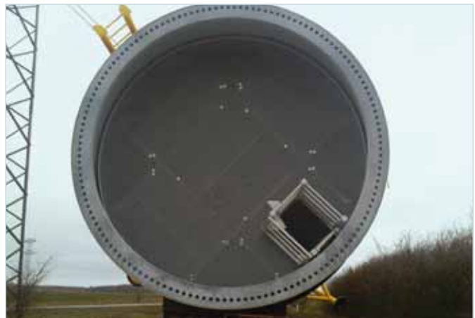
Intermediate level made from GRP-gratings
