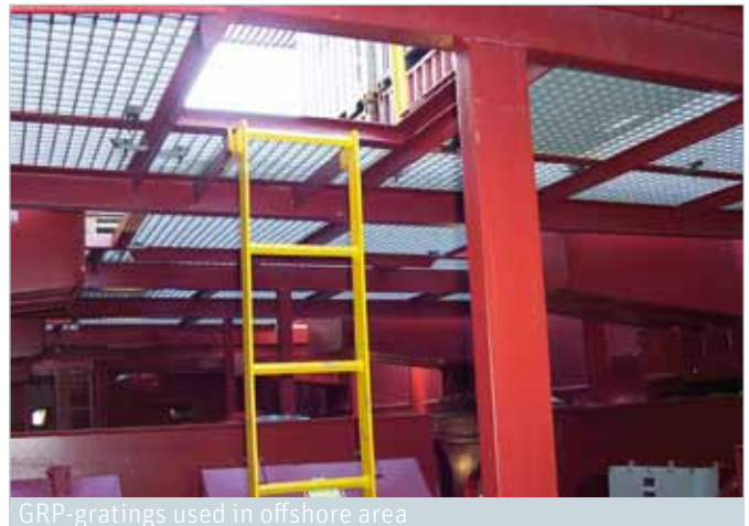
GRP-gratings used in offshore area
