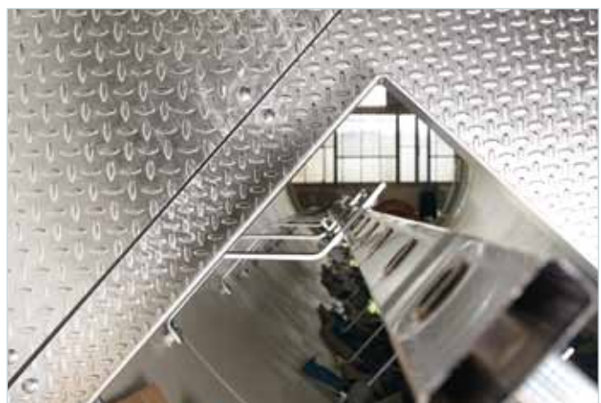
Intermediate level made from chequer plates
