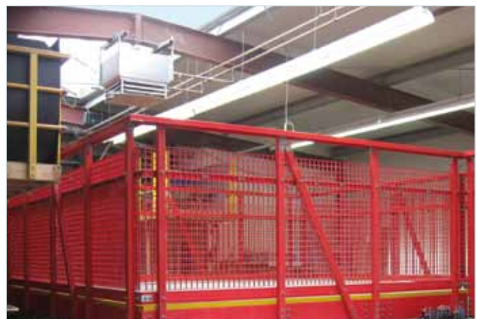
Temporary build at the plant
